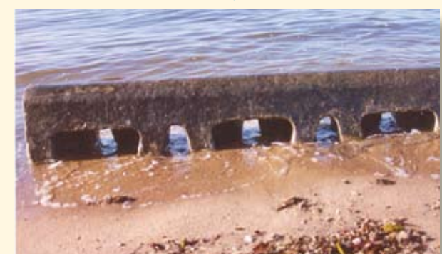
Terrapin Nature Area maintains 3 ft of sand accumulation, June 2004 (Installed July 1989)
