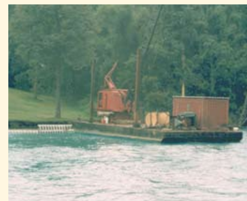
Barge installation is used when shore-based installation isn't practical
