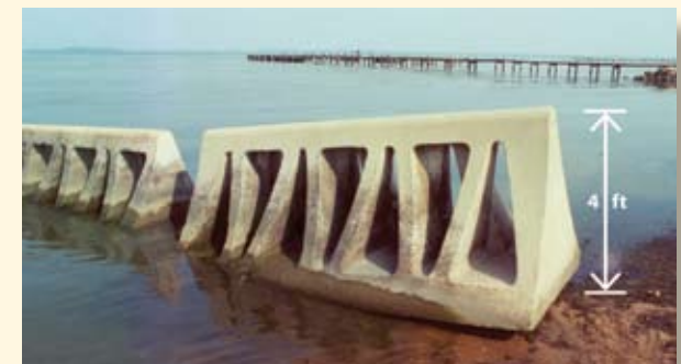
4 ft tall by 10 ft long; weight 9,100 lbs; high strength precast concrete with epoxy-coated reinforcing steel
