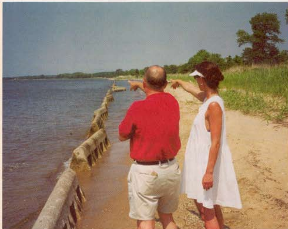
Picture of Terrapin Nature Area in 2004. Only 16 inches of the 4 feet in height of the Beach Prisms is visible, due to sand accretion.
